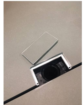
Line Drain Detail
